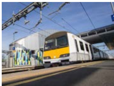
Southend Airport train station is just a short walk from the terminal.
